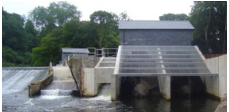
Photo shows part of Radyr weir (far left), the channel for eels and lampreys, the new fish pass and then the 2 Archimedes screws (far right) with the ancillary buildings for generating electricity and monitoring the fish behind.
